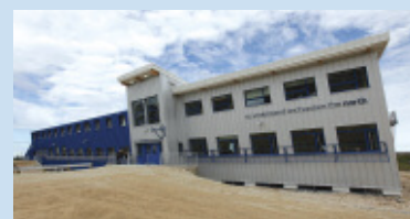
CNSC is a LEED® NC Registered Project that is targeting GOLD certification.
